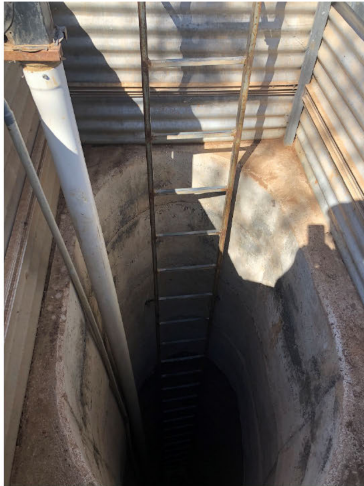
Image 3: Sophisticated mining claim shaft (concreted)
