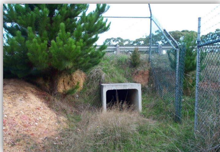
Figure 5-4 The fence on the right guiding koalas to the small koala underpass was left unfinished.
