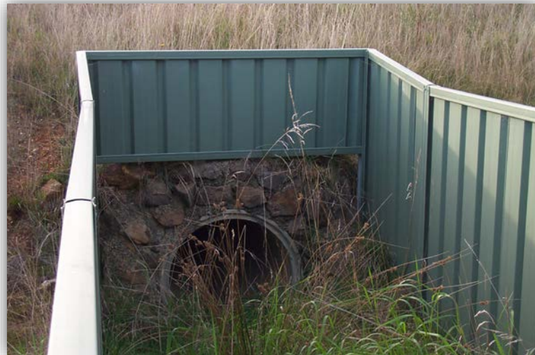
Figure 5-6 Second underpass—very narrow diameter, dark, continues for 60 m under the road.
