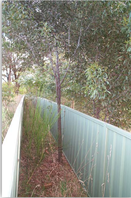
Figure 5-5 Labyrinth-like koala guide fence—overgrown with vegetation.
