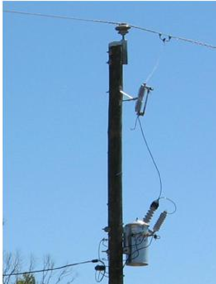
Figure 1.1: Typical SWER customer connection (Stanage Bay, Qld) [6].
