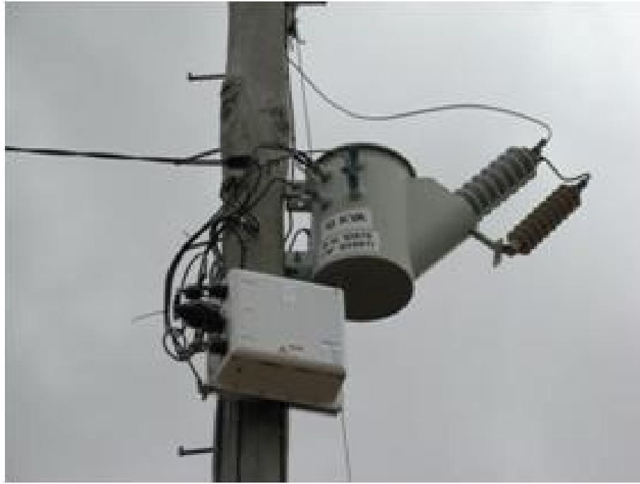
Figure 4.1: LVR installed on a SWER [7]
