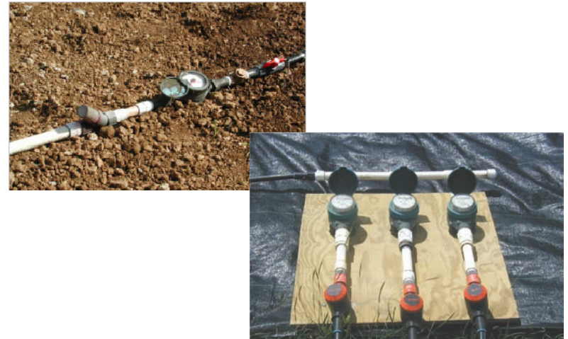
Figure 9. (l) Water meter installed near the field; (r) water meter and timer to control flow of irrigation water.
