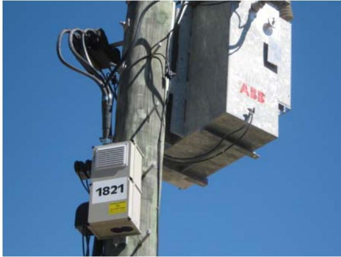
Figure 2. EDMI Mk10. PQ Meter 1821 in the field
