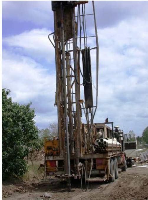
Figure 2.16: Drilling of piezometer wells
