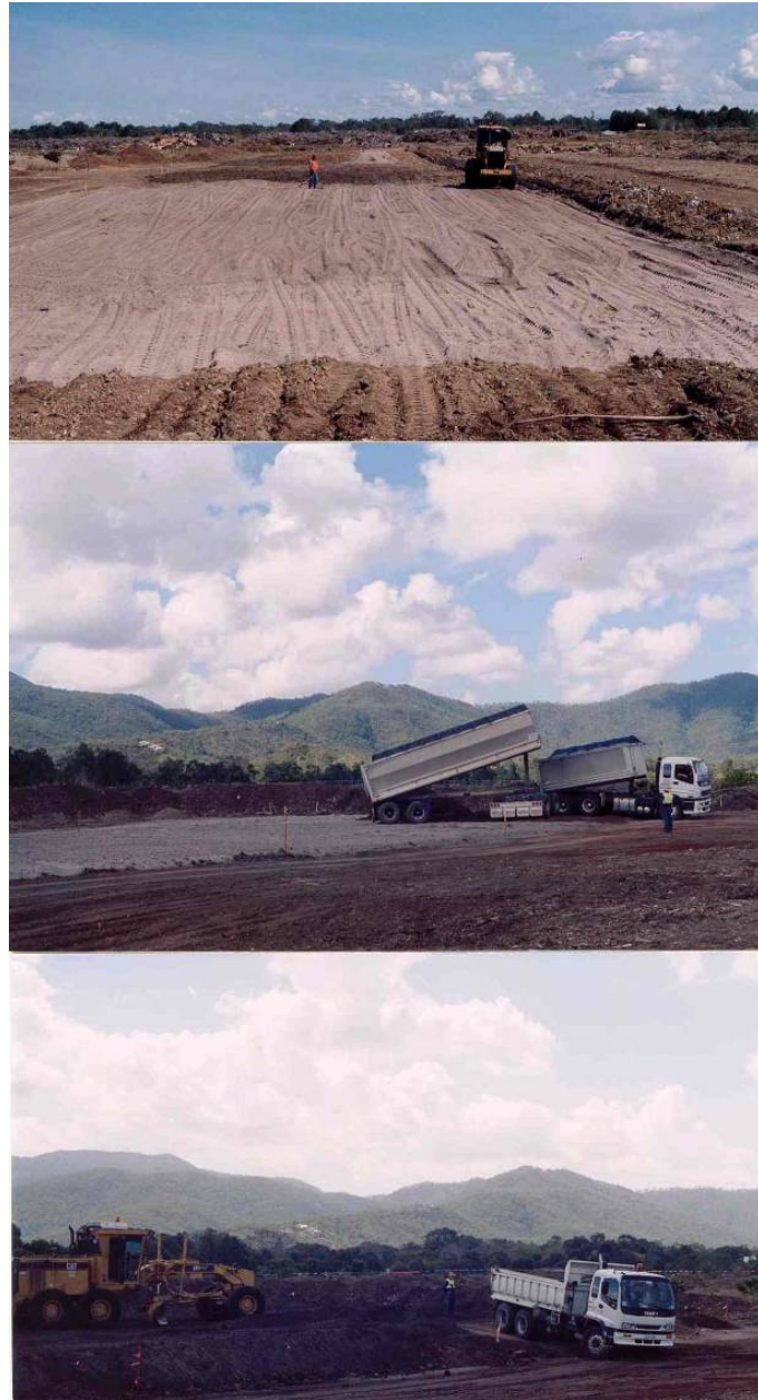
Figure 2.5: Various steps involved in constructing the Thick and Thin phytocaps (Photo: N. Ashwath)
