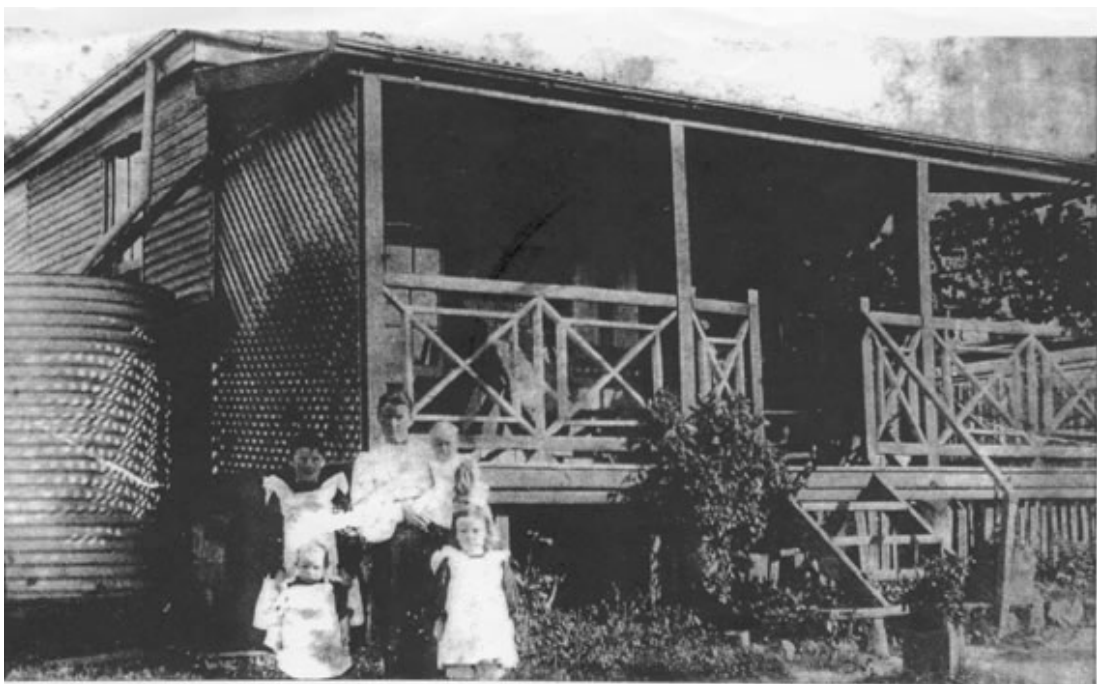
Fig. 3. Miner's family and cottage, note corrugated iron wall, lattice screen and in the ubiquitous style of the 1890s verandah railings of this design adorned houses, residences, hotels and the large office building at the mine.
