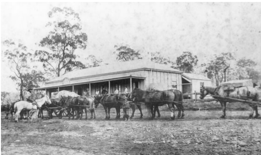
Fig. 10. Moongan Hotel, c. 1897. This structure shows a single line of rooms with french doors, a similar construction to the Sunburst Hotel. A detached kitchen and stables are at rear. These buildings contrast with the large Razorback Hotel, where rooms extend along a passage from front to back, (see Fig. 1).
