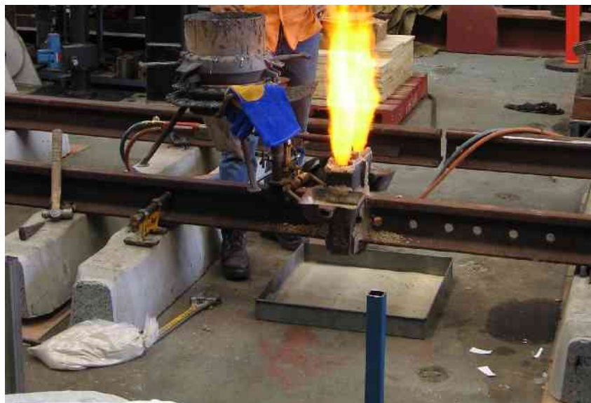
Figure 6.21. Track welding
