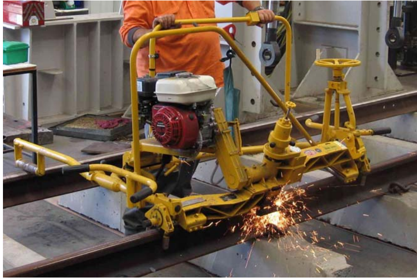
Figure 6.22. Track grinding
