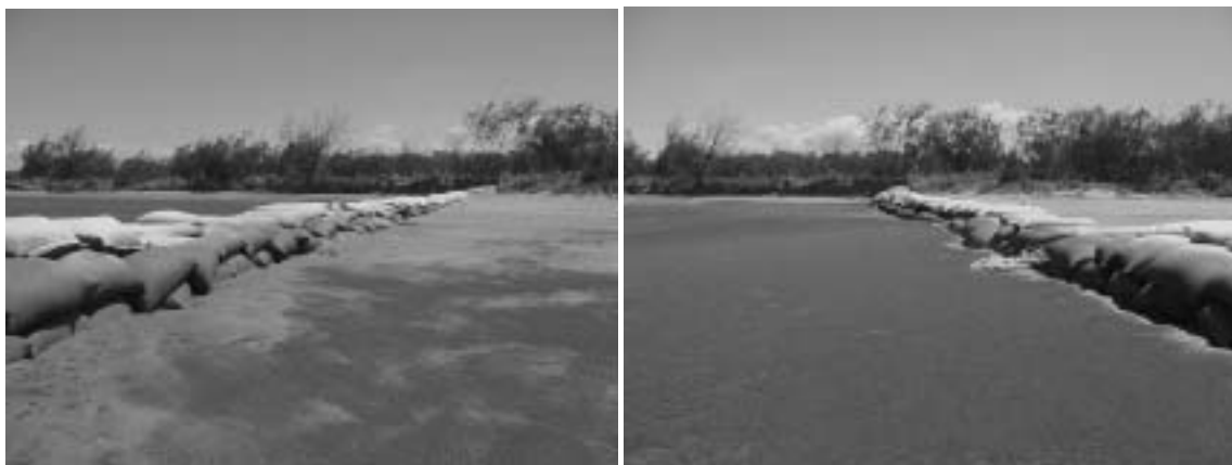
Figure 40. Geo-textile groyne on South Kinka, January 2002
