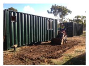
Figure 3.20: Soil distributed to cover the PVC buried tubes.
