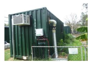
Figure 3.2: Experimental shed of the earth pipe cooling system.
