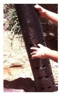
Figure 3.11: Manifold for vertical installation system.
