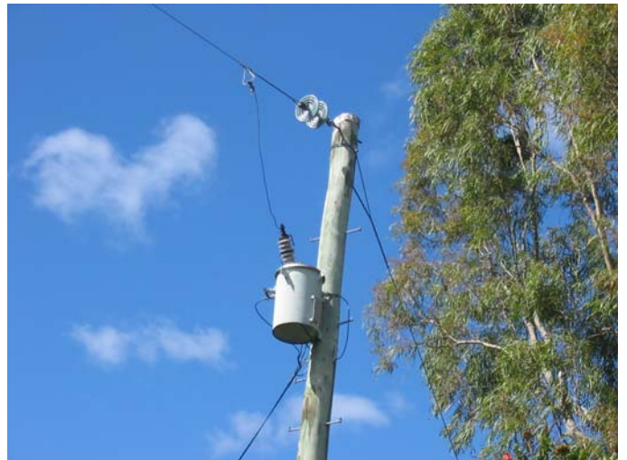
Fig 1. A SWER Customer Transformer, [8].
